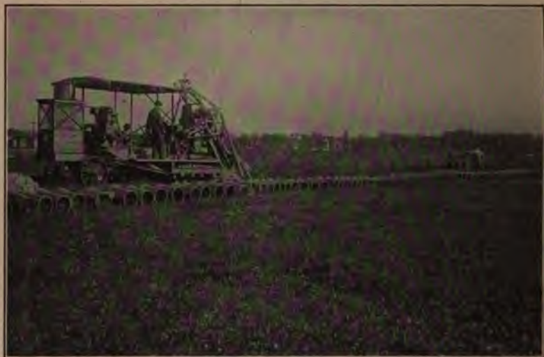
Austin Tile Ditcher.
